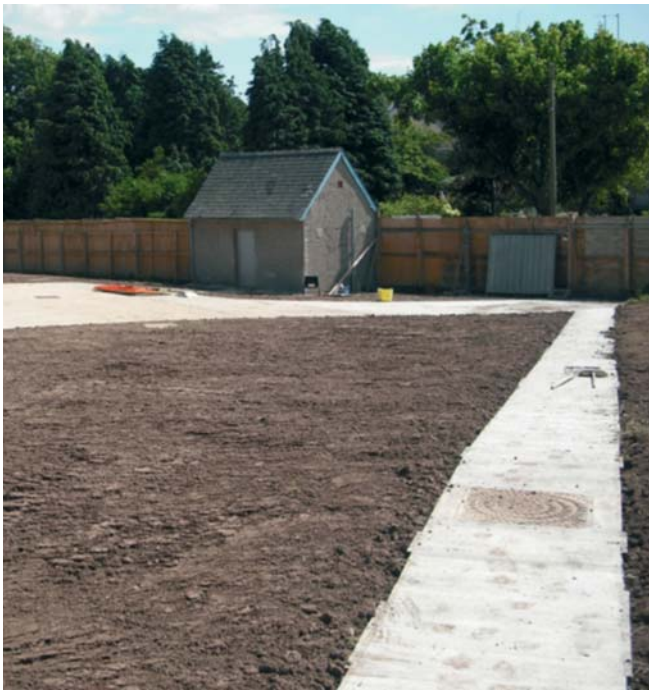
Steynton Nearing Completion
