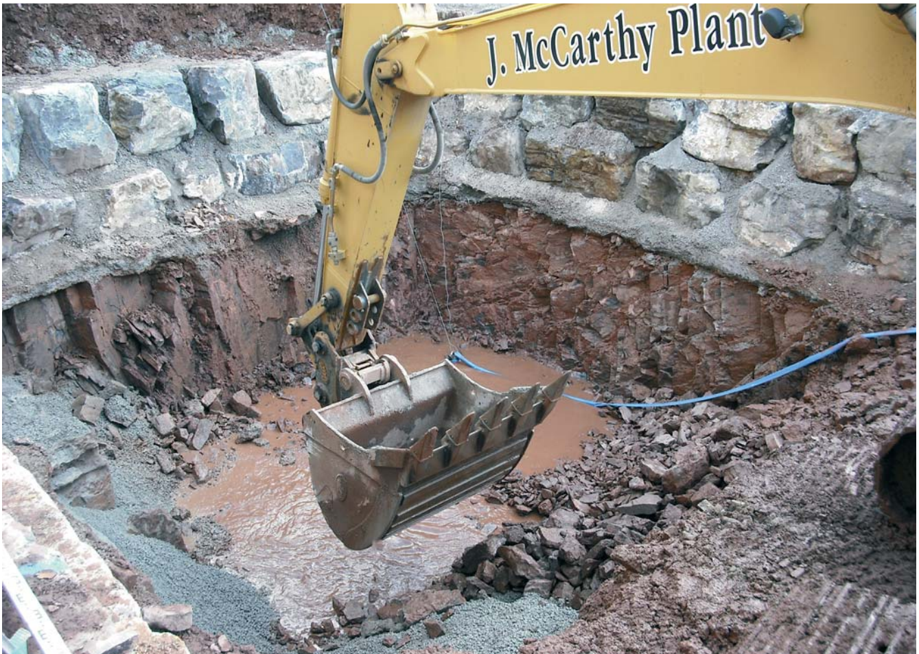
Excavation to Formation
