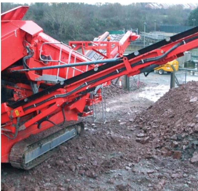
Screening at Merlins Bridge
