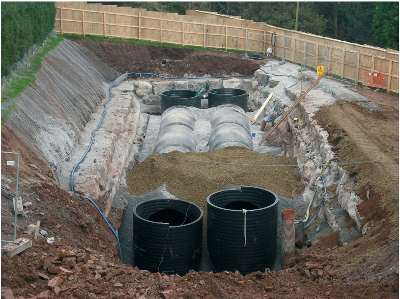
Processed Top Backfill Layer
